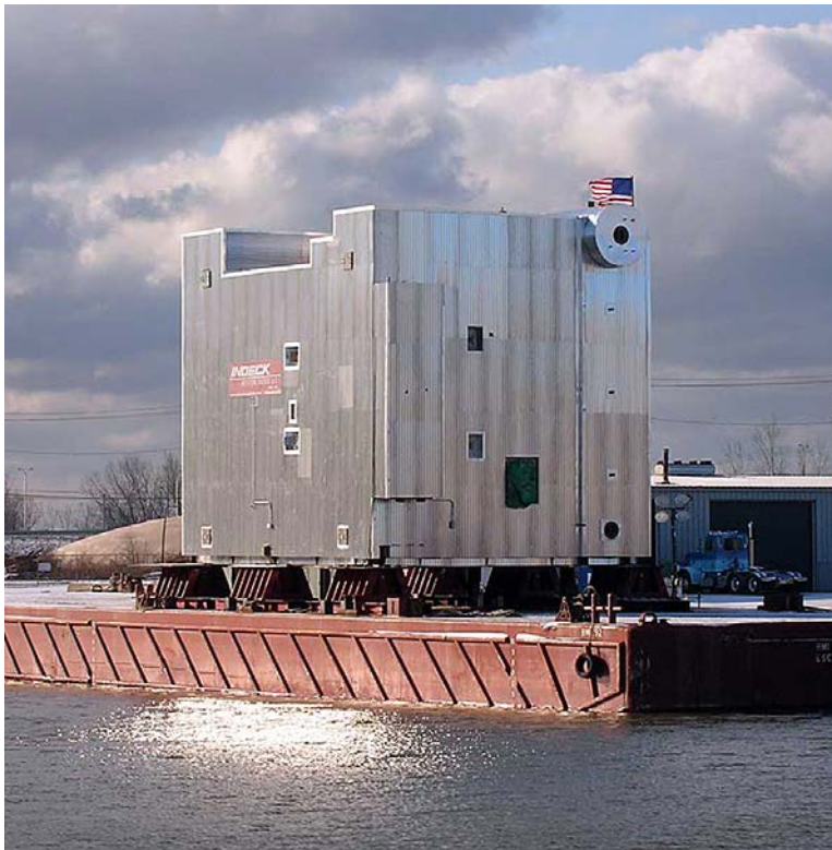
ArcelorMittal USA, Inc. installed an energy-efficient boiler at its Indiana Harbor Steel Mill that has the capacity to reduce carbon dioxide emissions by 330,000 tons annually. Photo from ArcelorMittal
