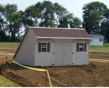
New Jersey builder Mark Bergman combined Building America building science know-how and a personal commitment to energy efficient construction to achieve energy savings of 46% over the Building America benchmark home. (Above) Wiring for the photovoltaic system runs underground from the sheds to the houses.
